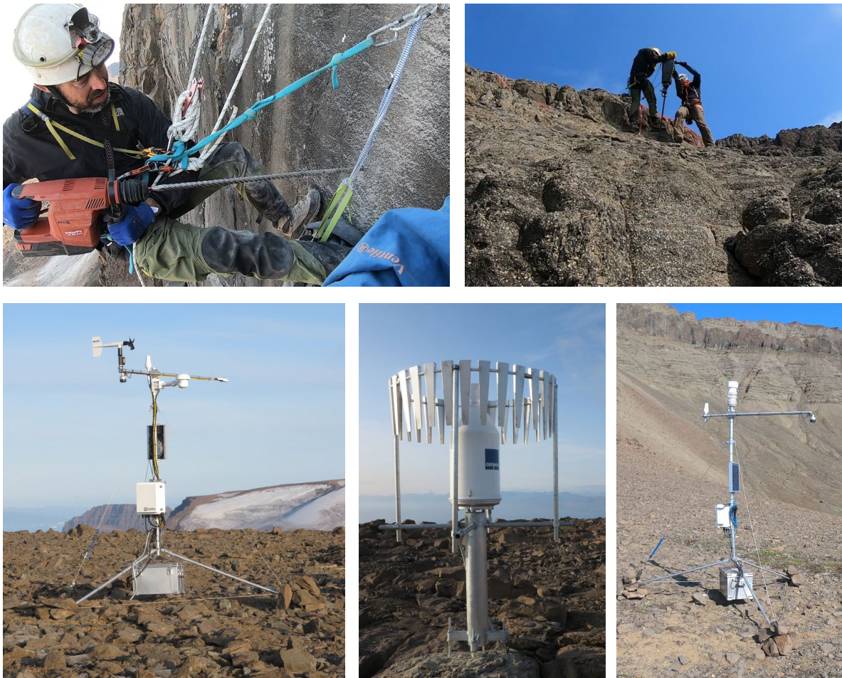
Figure 3: Drilling of bedrock boreholes for measuring the temperature of the rock wall down to 1 m and 2m depth (top left and top right, respectively). Automatic weather stations were installed at different elevations to measure near-surface weather (bottom).
